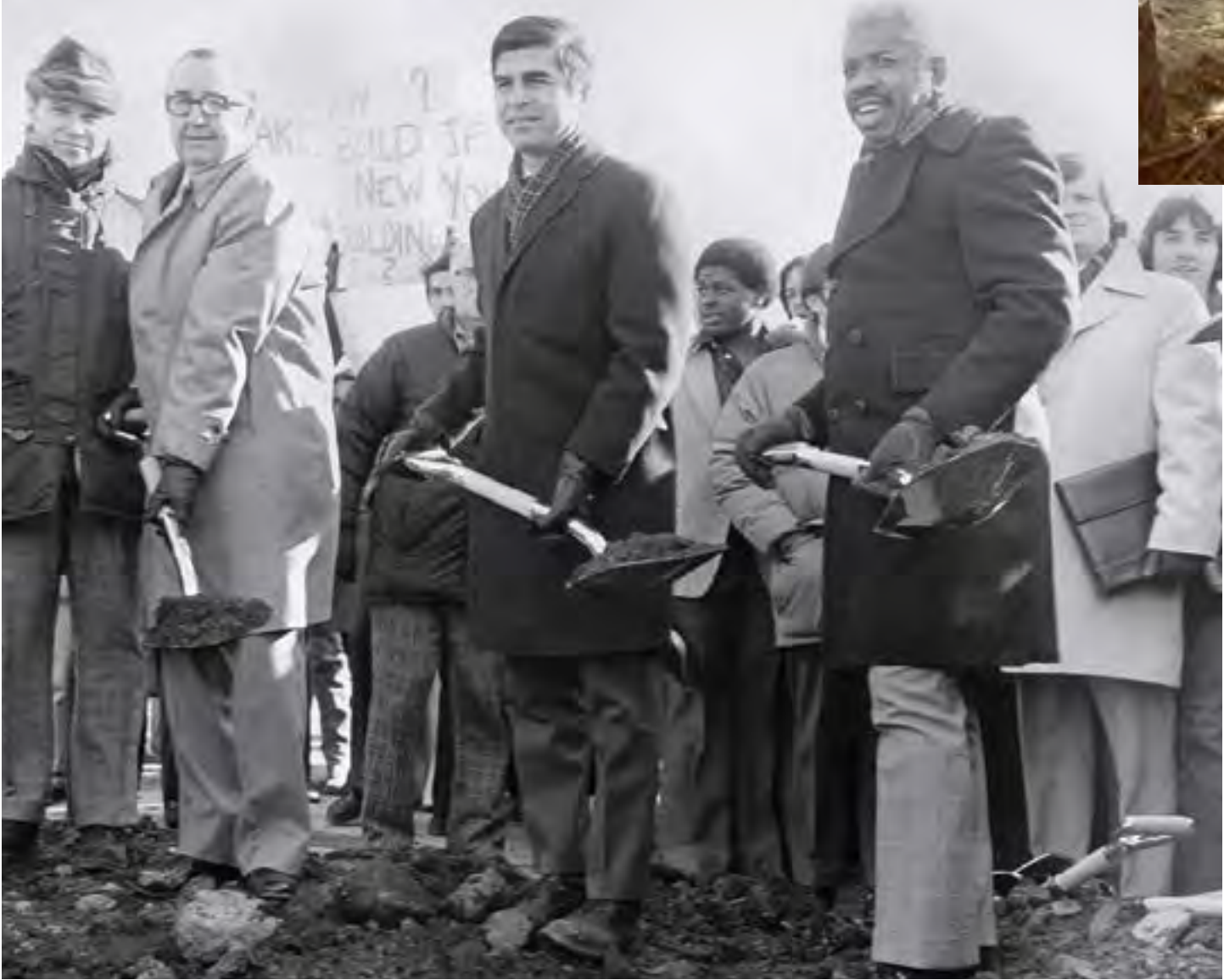
Dignitaries including College President Harold Shively (second from left), Massachusetts Governor Michael Dukakis (center) breaking ground for the College’s E-Building, constructed to meet the demand of increased enrollment. The E-Building opened in September 1979.
