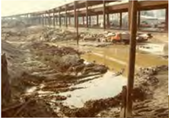
Construction of the Charlestown campus gets underway.
